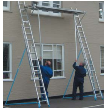
4. USING ERECTION TEES
