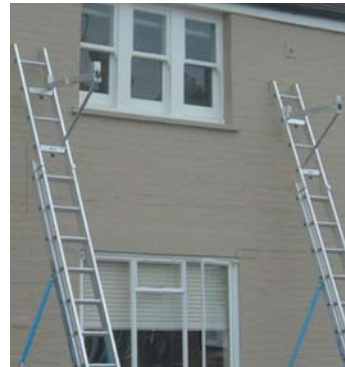
3. STAGING BRACKETS MOUNTED
