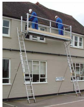
3. STAGING BRACKETS MOUNTED
