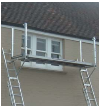
5. STAGING AND CORNER POSTS POSITIONED
