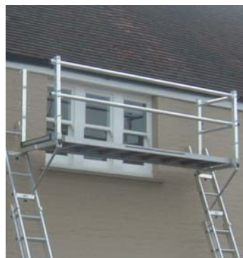
6. GUARD RAILS POSITIONED
